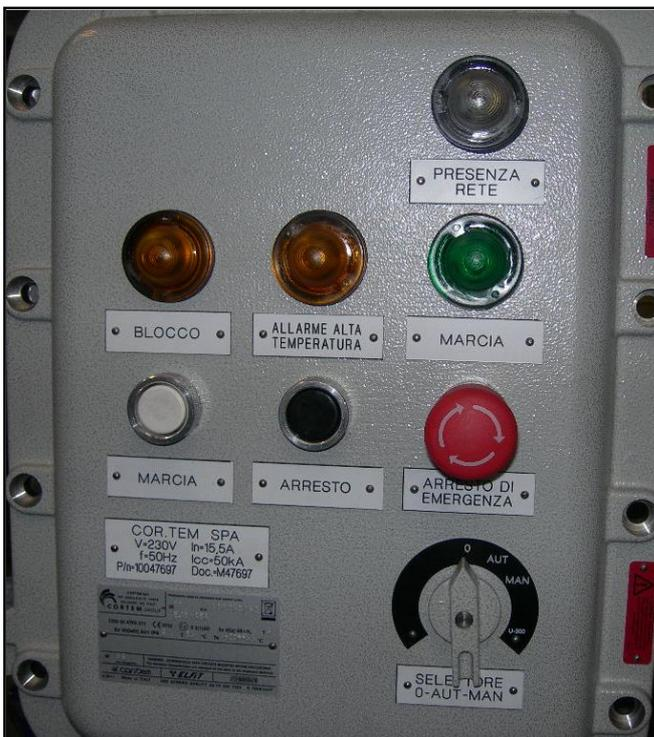
Fig. 1.1 View of control panel
