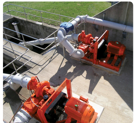
Permanently installed electric drive Dri-Prime pumps moving effluent from a secondary trickling filter to a chlorination chamber and then discharge.
