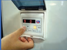
The microprocessor and the settings can be easily adjusted on the Display Panel. The microprocessor receives information and adjusts continuously the values to maintain the optimal energy gain from the Heat Pump.
