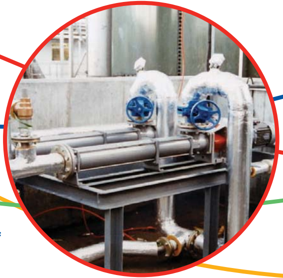
Pumping of slurry mix
